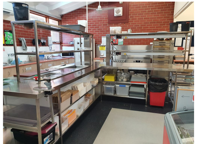
Above, the new shelving and bain-marie in the canteen.
